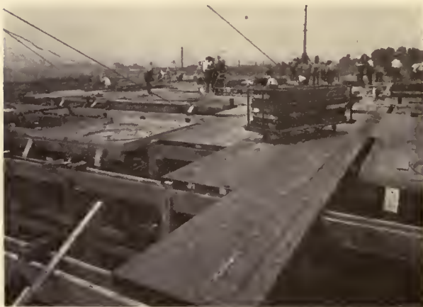
FIG. 5. PLACING THE STEEL PANELS
